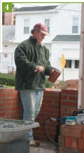
block walls up to floor level, and a large bump-out for the fireplace. **(Photo #1)** Rigid insulation was applied to the interior of the foundation walls to prohibit the cold passing from the ground, thru the block, and in to the inside slab which is their floor base. Mason Sonny Weaver laid the block walls up 8" wide from the footers up to slab height. Then he reduced the block size to 4" thick, creating a ledge around the inte-
