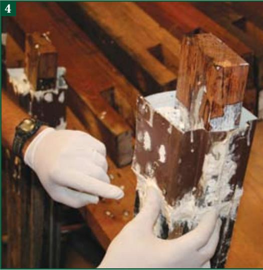
new pieces all laid out (Photo #5), it's easy to see how each solid piece of lumber was cut to create the mortises in the ends of the head and sill, and the tenons in both ends of the side legs (which Jim is holding). The tenons fit snugly into the mortises, and it all goes together a little like Lincoln Logs!
