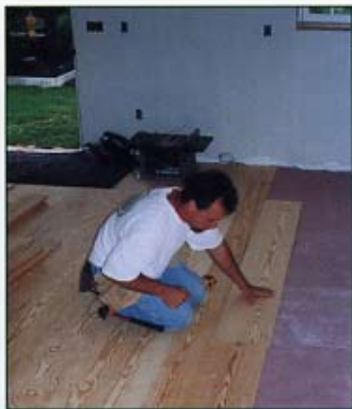
Rich is seen installing the wide, random-width, yellow pine flooring ▲
