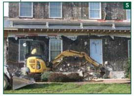
weightier stone facing. The crew from Haldeman's **Excavating very** carefully dug a narrow trench right against the house foundation, and also removed a massive concrete and stucco front-door stoop. (Photo #5) After we poured a reinforced footer, Sonny Weaver, Unique Masonry, then laid up a new block foundation up to grade. The Restore 'N More carpenters had already framed up the pent eave structure.
