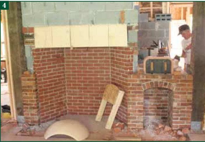
can see how the side and rear of the bake-oven dome is smack up against the Parlor fireplace, and the many flues are converging from all sides above him. It was just like the proverbial “stuffing 10 pounds of stuff into a 5-pound bag.”
