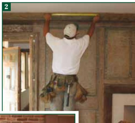
the hole above the fireplace proved that the room was eventually heated by a stove instead of the fireplace. But the original paneling clearly indicated how large the original fireplace opening was. Where no
